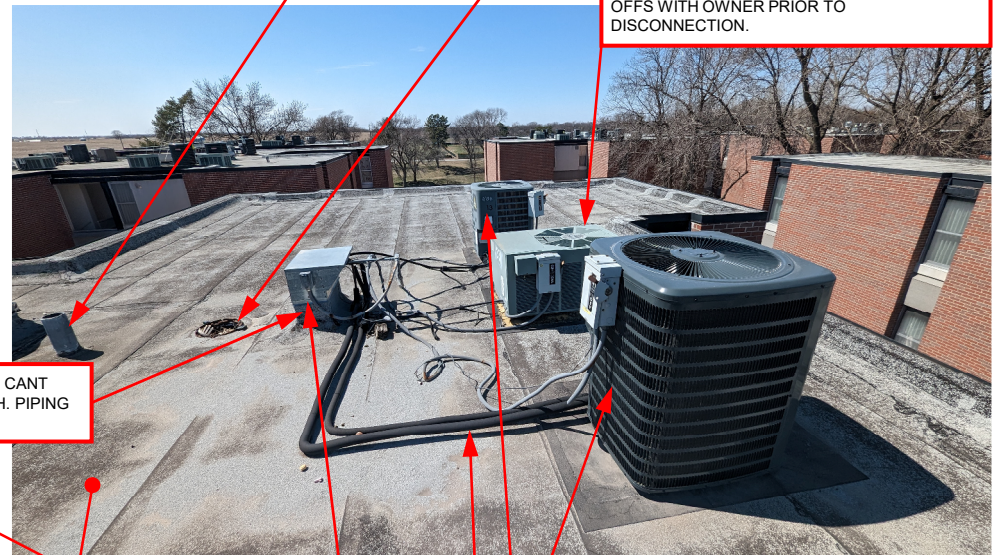
ROOF B (MATHEWS) - NORTHEAST
