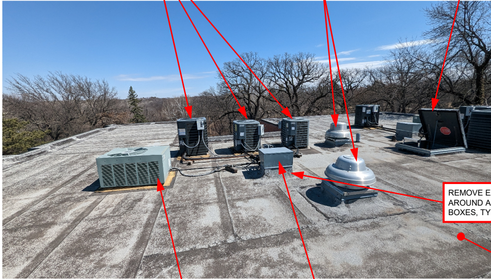
ROOF B (MATHEWS) - SOUTHWEST
