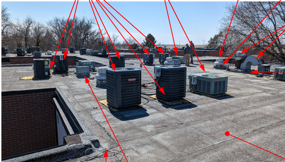
ROOF A (CLAYBURN) – NORTHEAST LOOKING SOUTH
